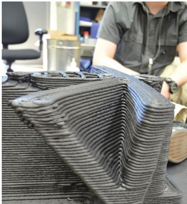
A close-up of part of the 3D-printed Strati.
